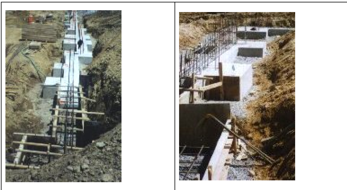
Photograph 4.1 – Shallow Spread Footings
