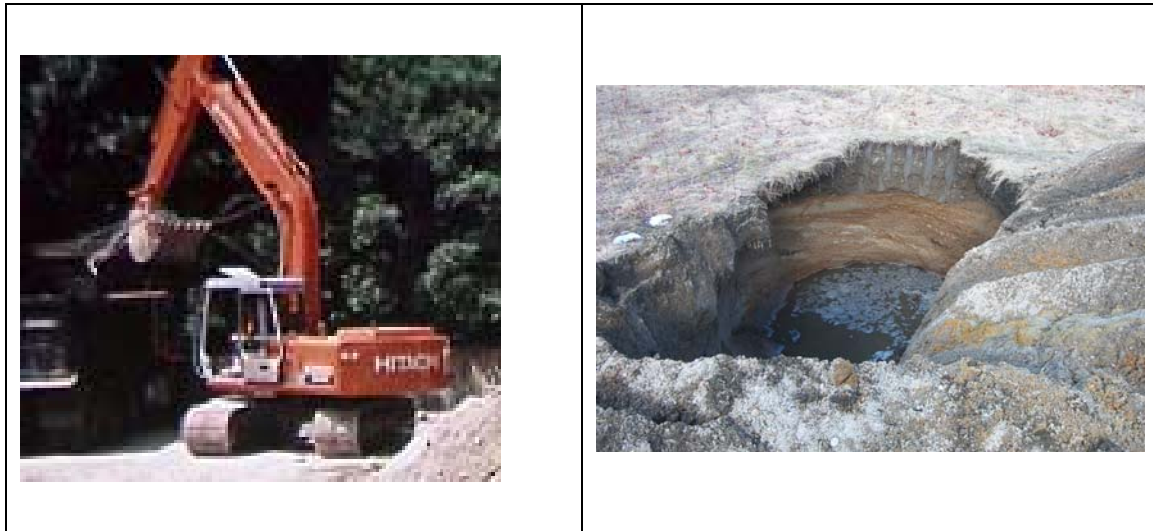
Photograph 2.1 – Test Pit Excavation
